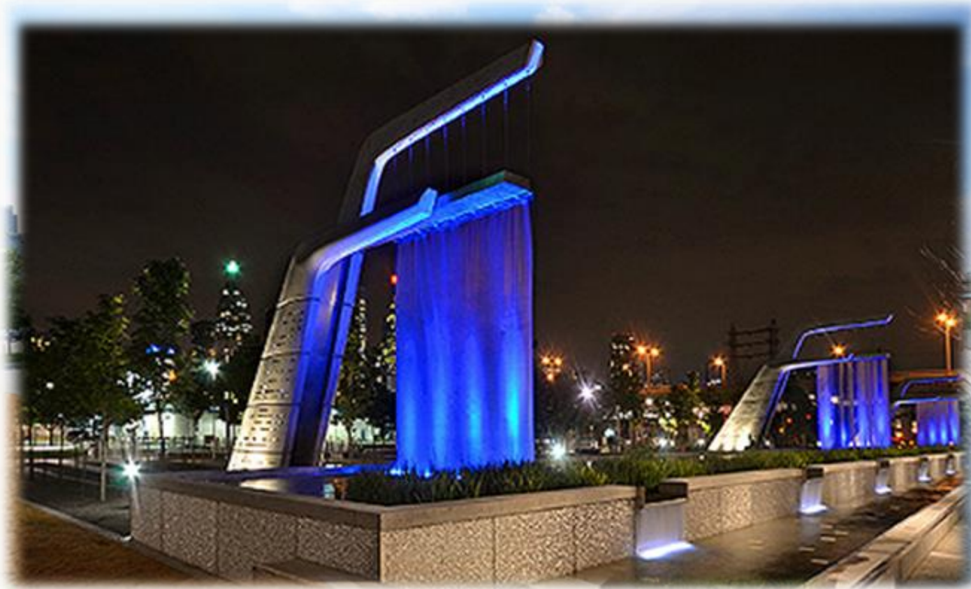
Storm water Treatment Plants
